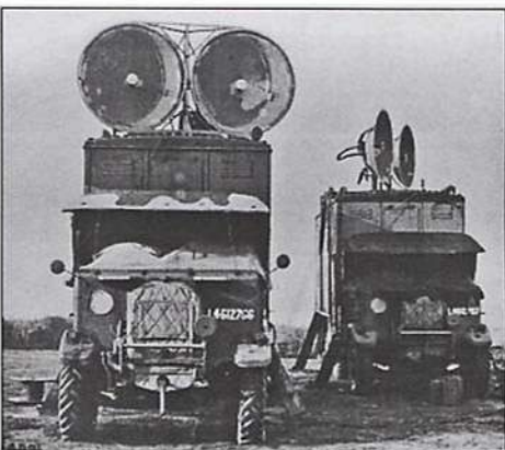
(Figure 10-6) Extemporised vehicles carrying early version of Wireless Sets No. 10
